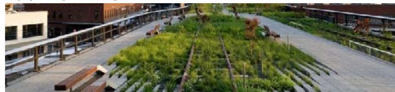
The High Line. Fuente: The High Line
